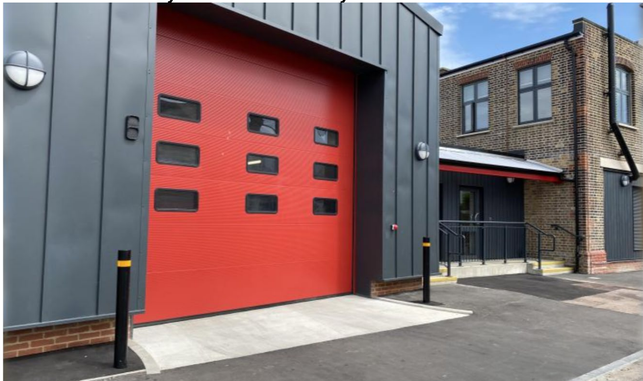
Pictured - The recently refurbished Shoeburyness Fire Station:
